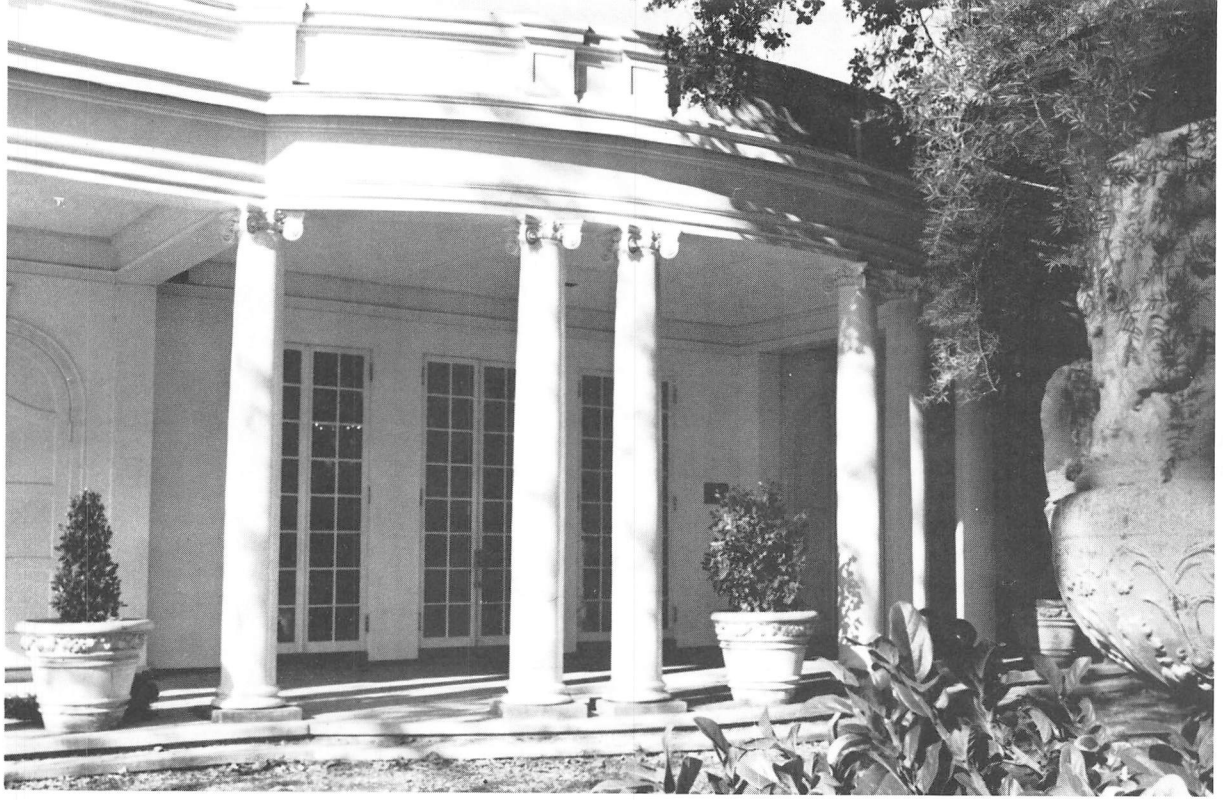
Exterior restoration of the Trianon was completed in the mid-70s after the building was moved onto its permanent foundation.
