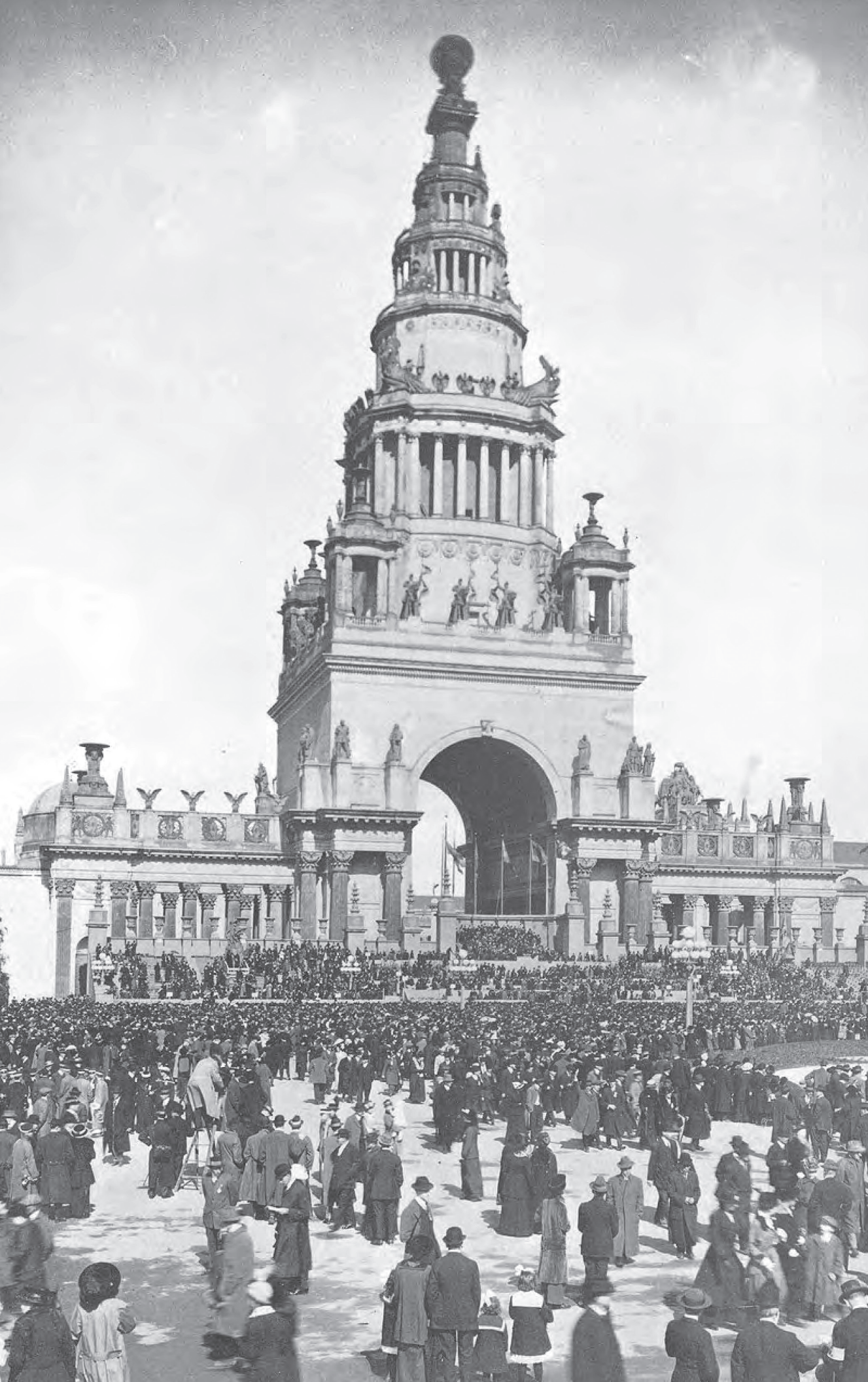
The Tower of Jewels on opening day, February 20, 1915. The Tower of Jewels was the dominating architectural feature of the Exposition standing 433 feet high and covering more than an acre of ground. Visitors entered through a vaulted entrance 60 feet wide and 110 feet high.
