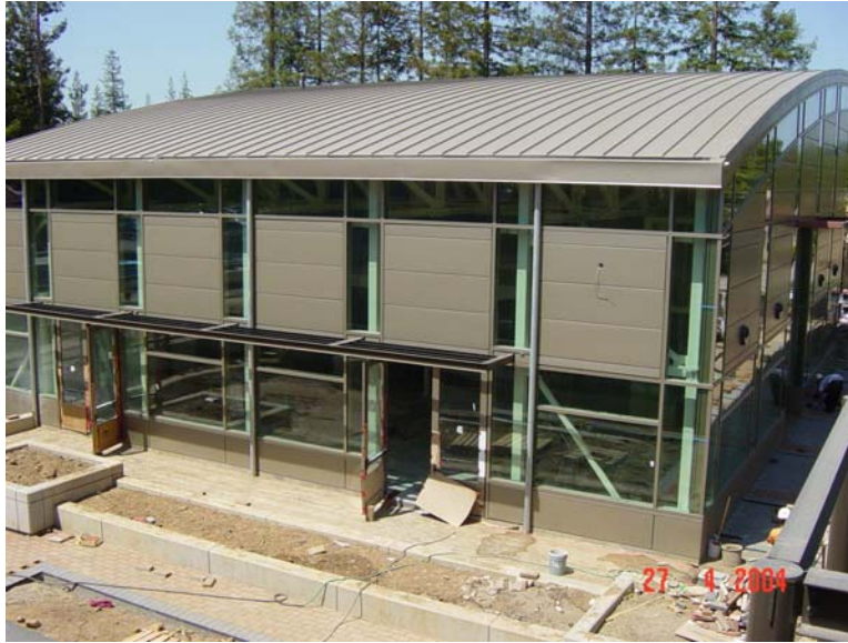
The Science Center under construction.
