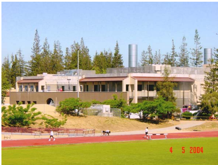
The Science Center under construction.
