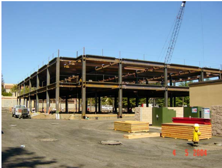
The new Student Services Center under construction.
